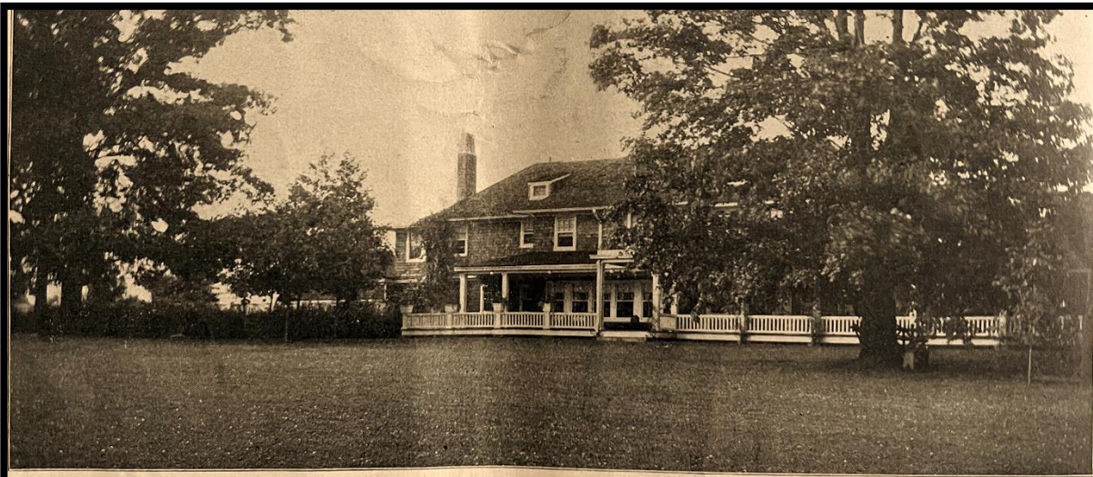
"Kingwood" is one of the largest estates in Lake County, comprising 600 acres of fertile valleys, uplands and forest. The Manor House occupies an elevated site affording entrancing views in all directions. "Kingwood" farm breeds Holsteins, Morgan Horses and Chester White Hogs. At the recent Lake County Fair, Kingwood Morgan and Kingwood Ethan Allan, two superb Morgans, won first prizes, and a Holstein Yearling Bull was awarded first prize.
