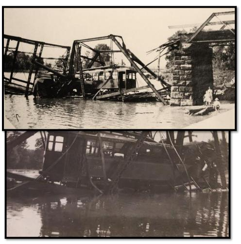
trailer, knocking it against a girder, which broke and weakened the bridge to such an extent that it fell to the level of the river. The bridge held at this point and prevented the car being plunged into 20 ft. of water. Eight of the injured were brought to the hospital here after
