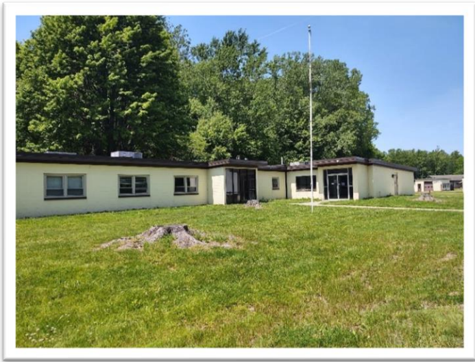
Control Area building consisted of a mess hall, admin. building, officers & enlisted barracks, van building and 3 20-foot towers.
