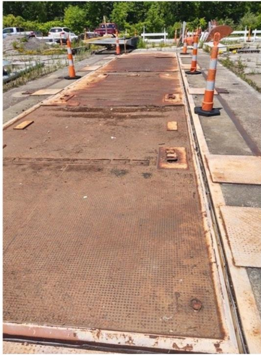
Painesville's CL-11 Nike Site launch bays.
